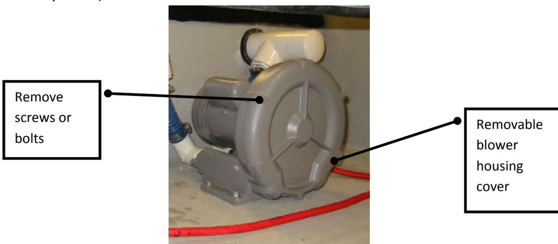
2.1.8. Remove all the screws or bolts that secure the impeller cover to the impeller housing. (See picture)
